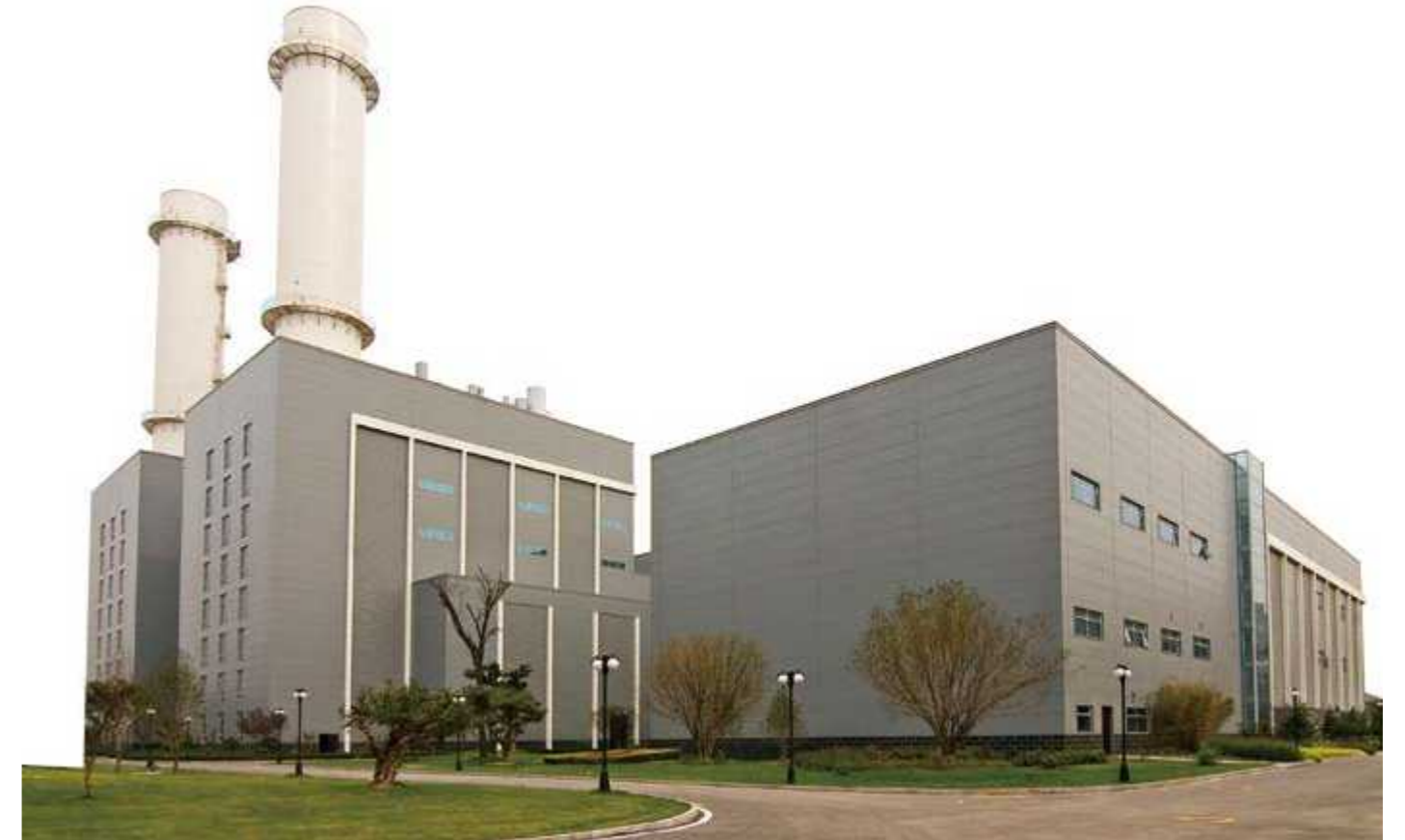
Beijing Taiyanggong 2×350 MW gas-fired CCHP Power Plant (Auxiliary Project of the 2008 Beijing Olympic Games)
