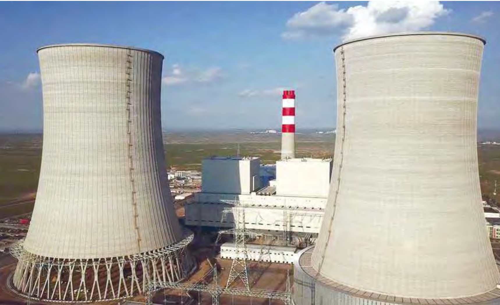
Guodian Ningxia Fangjiazhuang 2×1000MW Coal-Fired Ultra-supercritical Indirectly Air Cooling Unit
