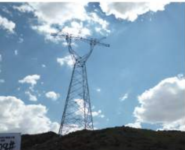
BNC9铁塔组力整体
